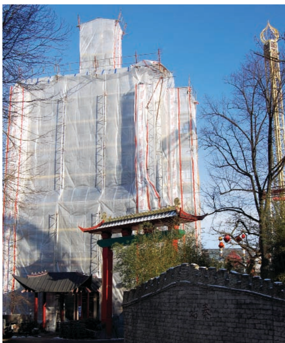
Throughout the winter 2010, the Chinese Pagoda is being renovated.
